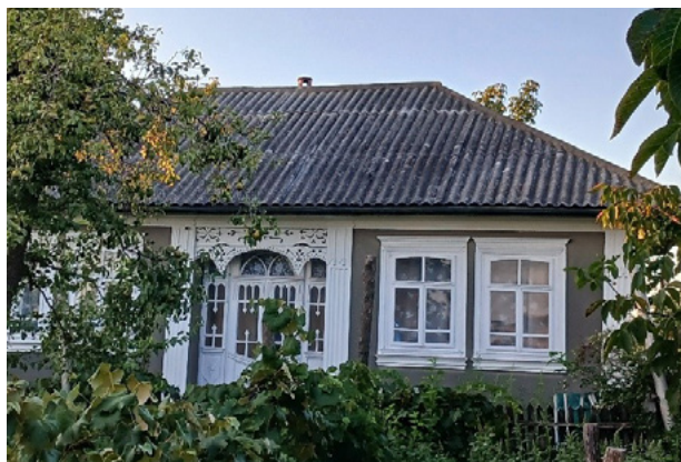
Image 12. Old renovated house. Northern region
